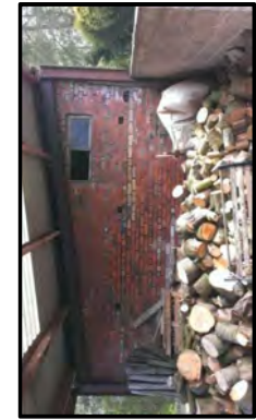
North Elevation (brick / blockwork to be removed existing steel structure to be retained)
