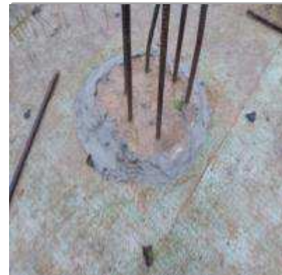
Tanking detail completed around pile cap.
