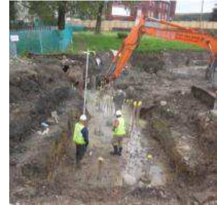
Blinding works to pile bases.
