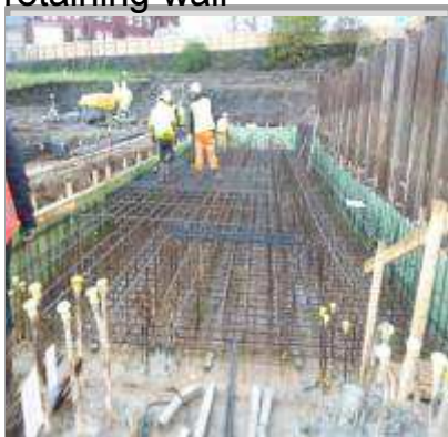
Steel reinforcement to retaining wall base
