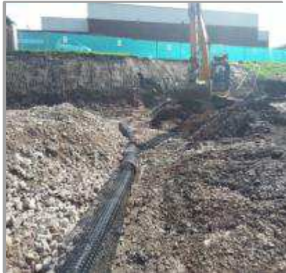
Geo-Grid being laid below 6f2
