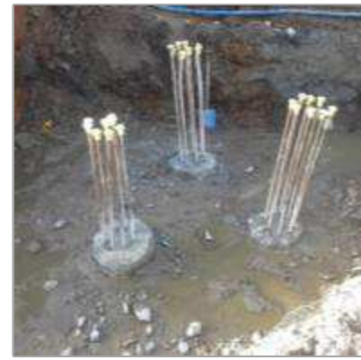
Cropped piles ready for blinding and integrity testing.
