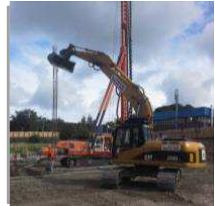
Steel cage being transported to pile location
