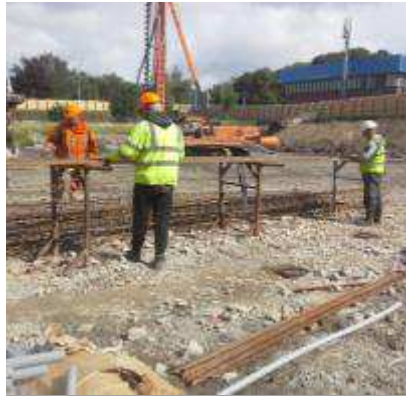
Steel cages being prepared
