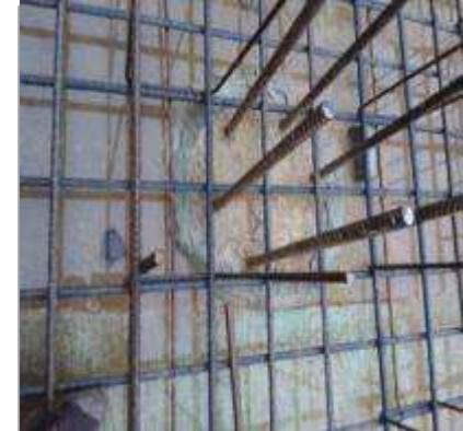
Beginning of mesh reinforcement being installed .
