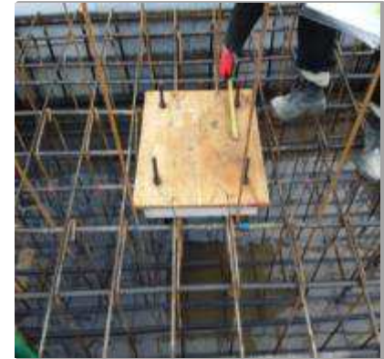
Connection bolts fixed in place.
