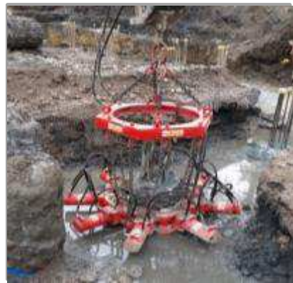
Concrete pile being cropped.
