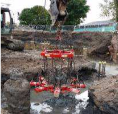
Concrete pile being cropped.
