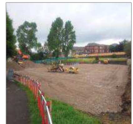
Finished level of piling matt
