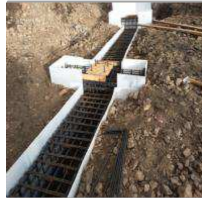
Steel pile caps and beams ready for concrete.
