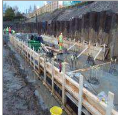
Timber shuttering for retaining wall
