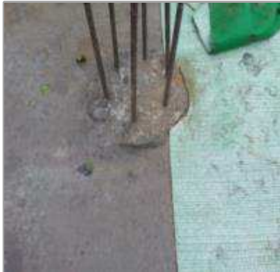
Tanking detail installation within retaining wall
