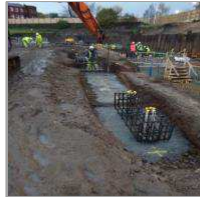
Pile caps and beams exposed
