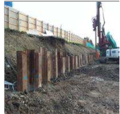
Installation sheet piles.
