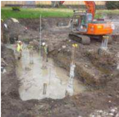
Blinding works to pile bases.
