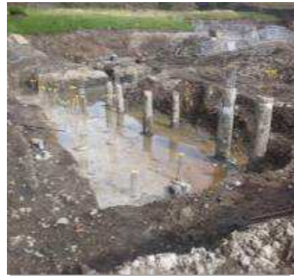
Reduced stepped level dig to expose piles.
