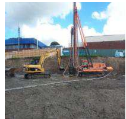
Piles being concreted in
