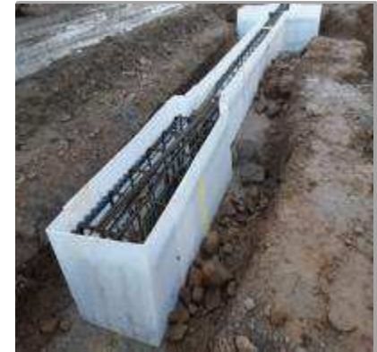
Formwork installed two pile caps and beams
