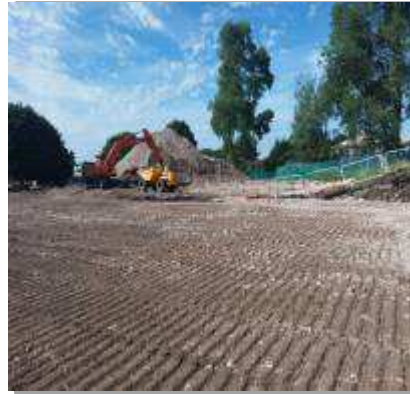
Levelling Piling matt
