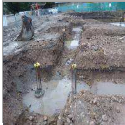
Cropped piles ready for steel cages
