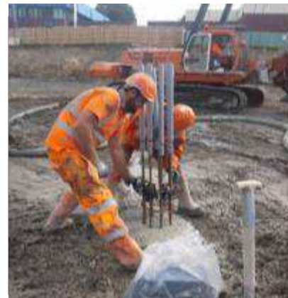
Pile reinforcement cage being installed.
